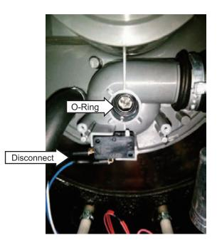
**Note:** Ensure the O-ring is retained in the sump before reassembly.
